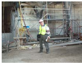
Consulting at Golden Gate Bridge Retrofit
